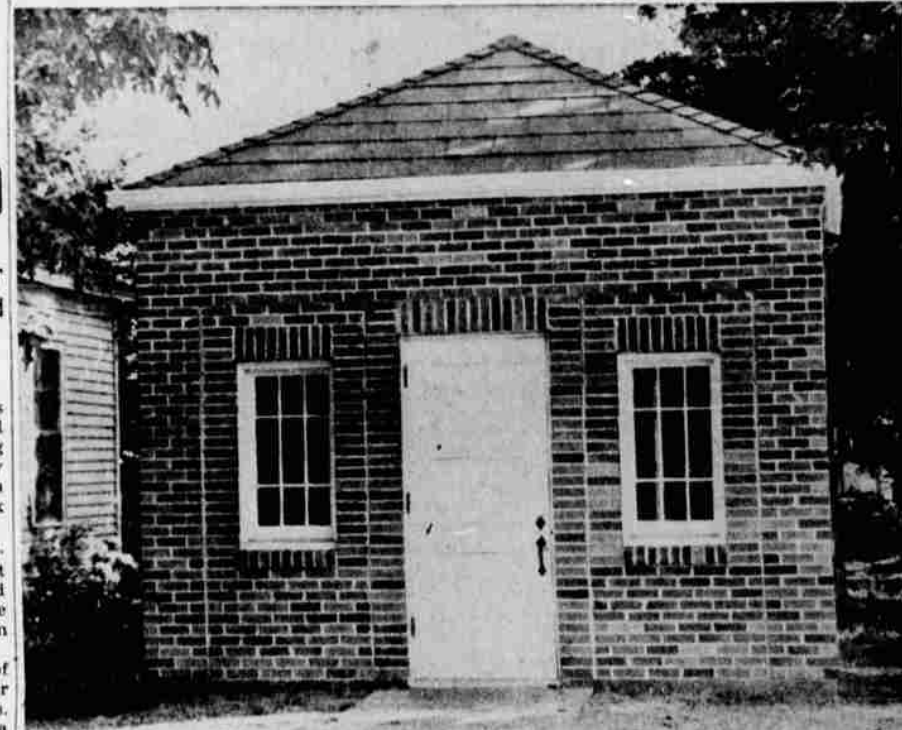
The new building (above), has been constructed at Jacksonville to house the Jacksonville dial equipment.
