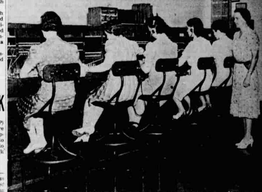
A portion of the new combined information and long distance switchboard in the enlarged telephone building is shown above. Miss Myrta Otterdale, chief operator, standing. The operators, from left to right, are Edythe Gault, Gladys Flora, Wilma Lemmon, Lucille Merrifield, and Elva Hamilton.
