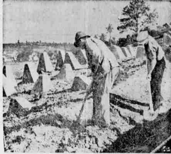
THEY SHALL NOT PASS, decided Germany, thinking of enemy tanks, and so teeth-like concrete blocks designed to rip off tanks' caterpillar treads supplement the Limes steel and stone defenses. The fortifications, built to match France's Maginot line, is to be finished this winter
