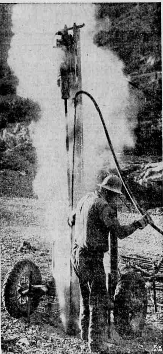
MAN-MADE GEYSER spouts rock dust at the site of a temporary diversion channel—part of the Shasta dam project on the Sacramento river, California. The workman has turned a stream of air into the hole to clear it of rock dust. The hole he is drilling is to be used to blast out rock in the canyon, where the dam is being built by the U. S. bureau of reclamation.
