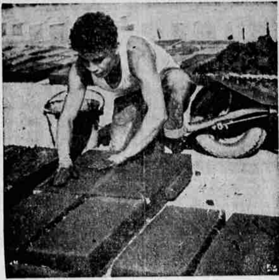
BRICK BUILDER Carlos Martinez, CCC youth who is helping restore mission near Lompoc, Cal., to its 19th century glory, carefully molds adobe bricks for use in the restoration. Wooden mold gives the bricks their shape. One minor tragedy among the CCC brick-makers was the loss of some 5,000 adobe bricks left in the sun to dry; a rainstorm melted them all.
