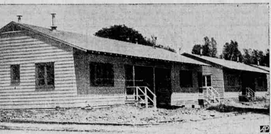
START OF SHASTA DAM on the Sacramento river, key unit of the $170,000,000 Central valley project has "boomed" towns, resulted in construction of houses (above), for use of government officials, engineers, etc. The dam, which will harness flow of Sacramento, McCloud and Pit rivers, will be executed only by Boulder in height and by Grand Coulee in mass concrete. It is to be 560 feet high, three-fourths of a mile across at top, and will back up lake 35 miles long.
