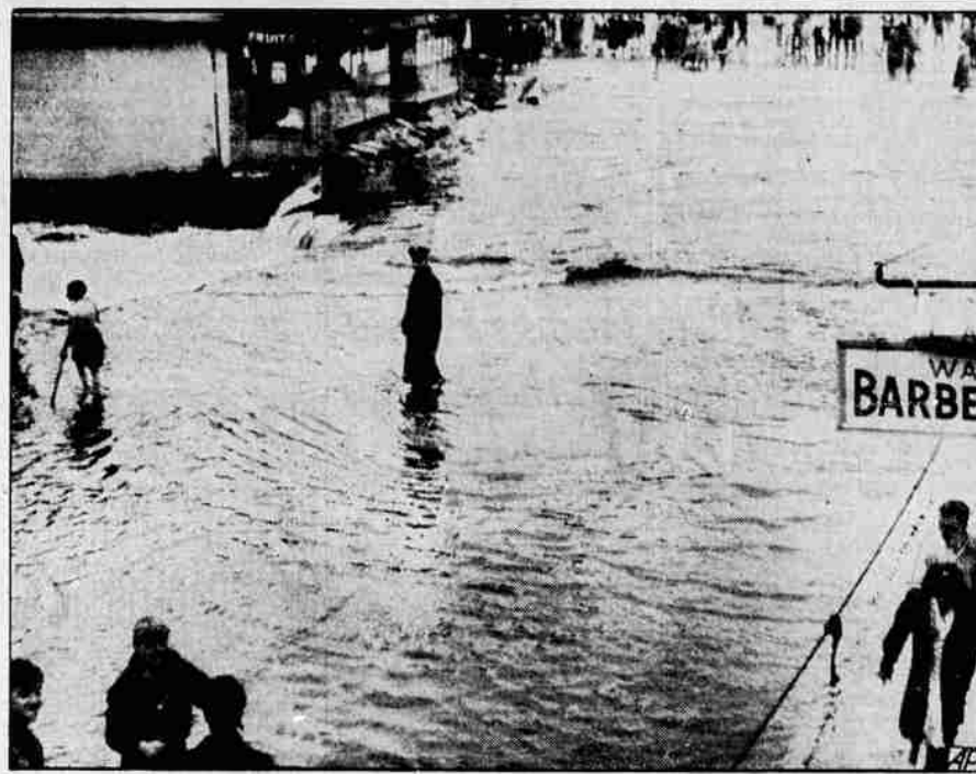
A week of solid rain produced this scene on the main street of Milford, Mass., where flood waters swept through the heart of the town and caused high property damage. Twelve lives were taken by the ruinous floods.
