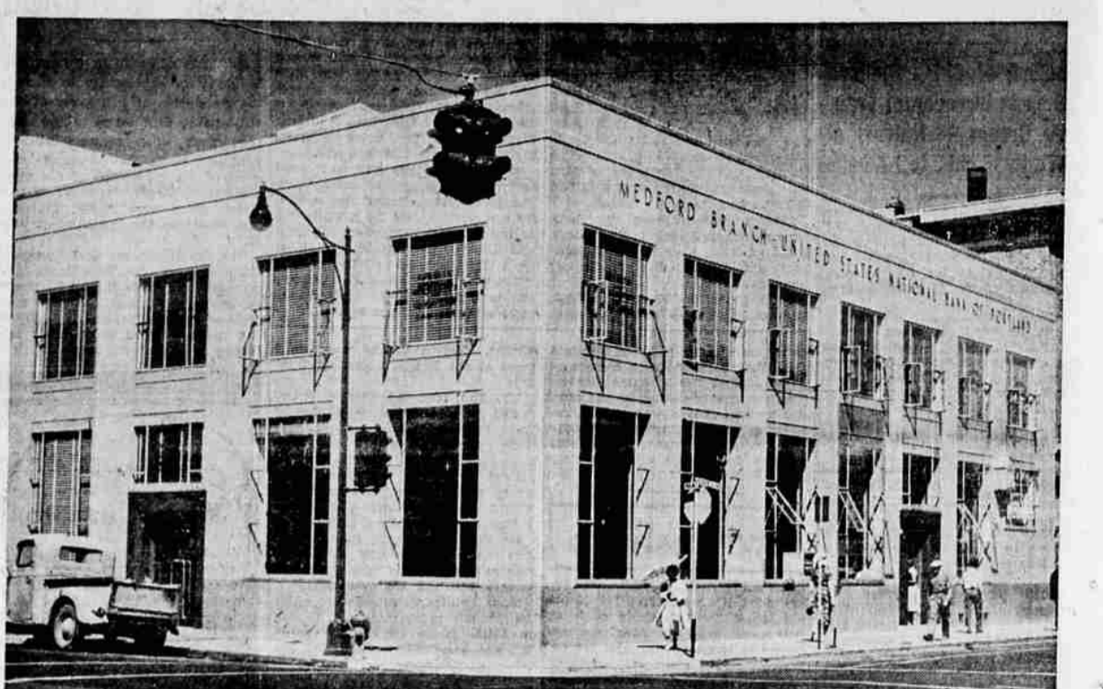
Two buildings at the corner of Main street and Central avenue were remodeled in completing this handsome, new home of the United States National Bank. The building, faced with pink Tennessee marble, has a 50-foot frontage on Main street and 80-foot frontage on Central avenue. Elmer Childers, well-known Medford contractor, supervised the complete modernization program. A public reception will be featured Saturday afternoon between the hours of 3 and 9, so that southern Oregon people may thoroughly inspect this attractive bank building.
