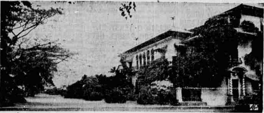
AGAINST 'McNUTT'S PALACES,' as he termed proposed new residences for Philippine high commissioner did Rep. Albert J. Engel speak, as House took up Army appropriation bill containing an item of $750,000 for 76-room winter home and 43-room summer home for the commissioner. Above are views of Manila residence which has been used by Commissioner Paul V. McNutt. He recently testified that house he had been renting for $6,600 yearly would no longer be available.
