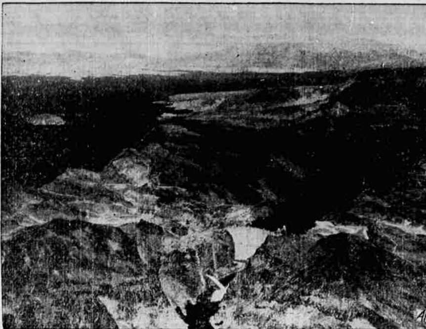
A MAN-MADE GIANT BECOMES A DWARF beside nature's rugged mountains and canyons. Mighty Boulder Dam, greatest structure ever built by human hands, appears tiny indeed nestled in Black Canyon of the Colorado river. Behind its 726-foot wall has formed Lake Mead, 115 miles long and containing 15,250,000 acre-feet of water, enough to cover West Virginia a foot deep. Capacity of the lake is 30,500,000 acre-feet.
