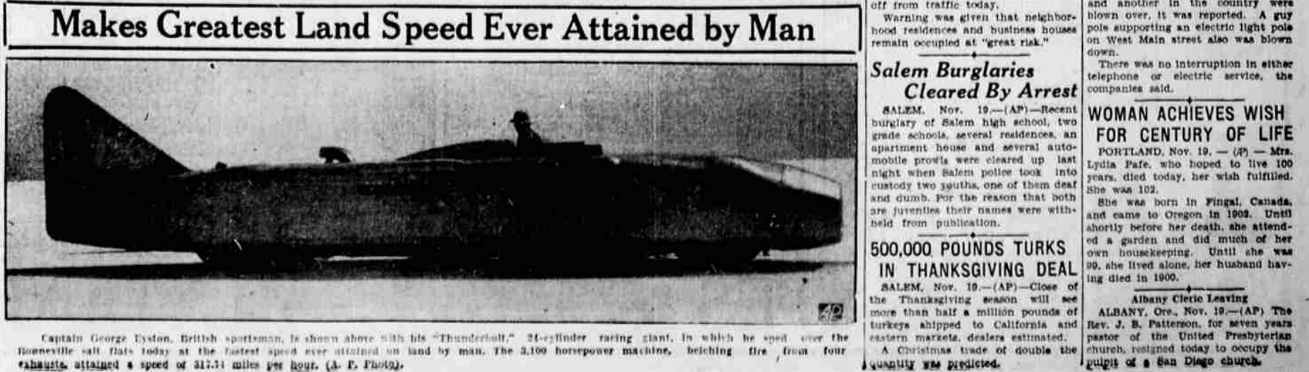
Captain George Eyston, British sportsman, is shown above with his "Thunderbolt" 24-cylinder racing car, in which he sped over the Bonneville salt flats today at the fastest speed ever attained on land by man. The 2,100 horsepower machine, belching fire from four exhausts, attained a speed of 317.42 miles per hour. (A. E. Photo.)
