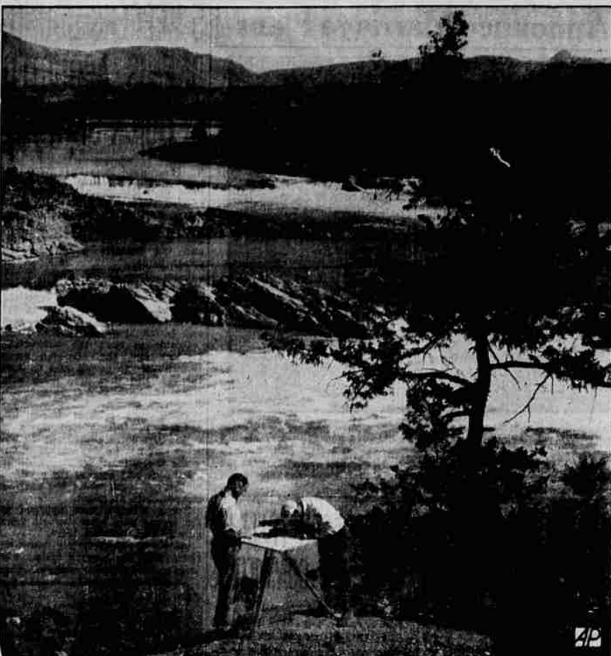
STILL WATERS WILL RUN DEEPER At Kettle Falls on the Columbia river, 110 miles above Grand Coulee dam when the mighty reservoir is completed, backing up an inland sea 151 miles to the Canadian border. Here is a plane table party surveying the reservoir basin. A continuous head of water will be supplied dam turbines generating power and water sufficient to irrigate 1,200,000 acres of desert will be available.
