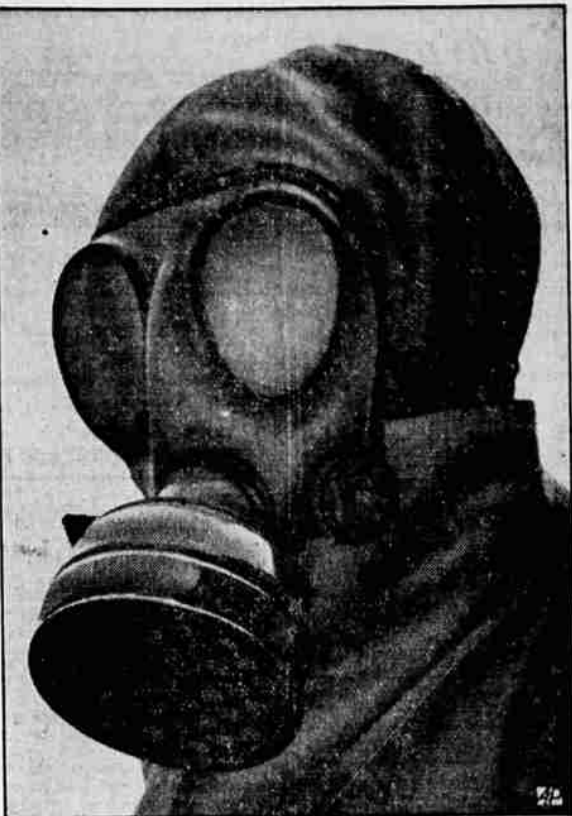
DOUBLE TROUBLE can hold no terrors for this wearer of the "Man from Mars" headgear. His aviator's helmet protects him high above the earth, while his mask safeguards him if he lands in an area under injurious attack. Austrian engineers developed the combination.
