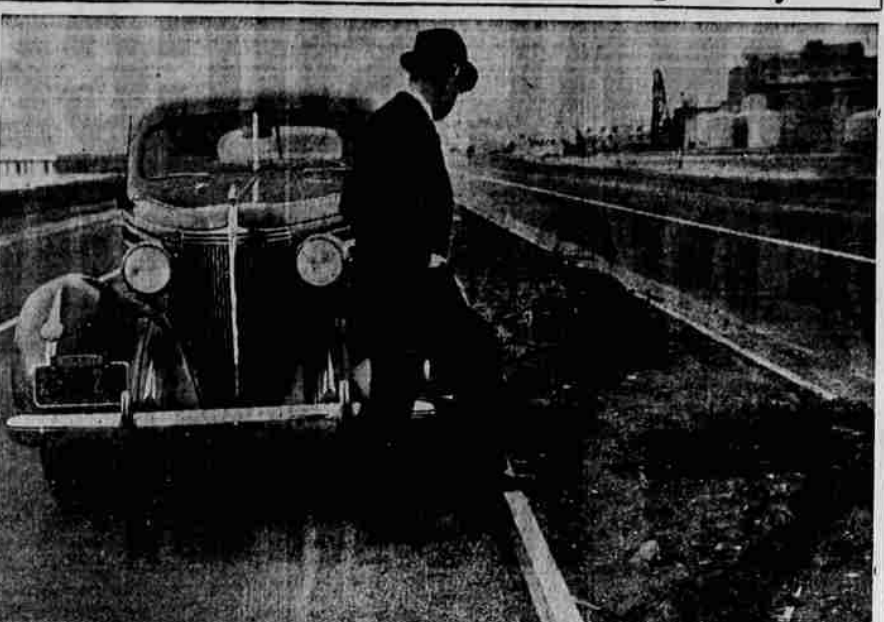
Here's the divided highway on the Berkeley approach to the San Francisco Bay bridge which has been termed an "ideal" for highway engineers to shoot at in future construction by both the Northern and Southern California automobile clubs. The wheel tracks show how difficult it would be for a head-on collision to occur, since the jolt of going over one curb and through the soft dirt is almost a sure guarantee of awakening a dozing driver. Safety features of the Nash Ambassador Six, which has paused beside the highway safety strip, include overdrive hydraulic brakes, finger-tip steering, all-steel body with safety steel top, and safety glass in all windows.
