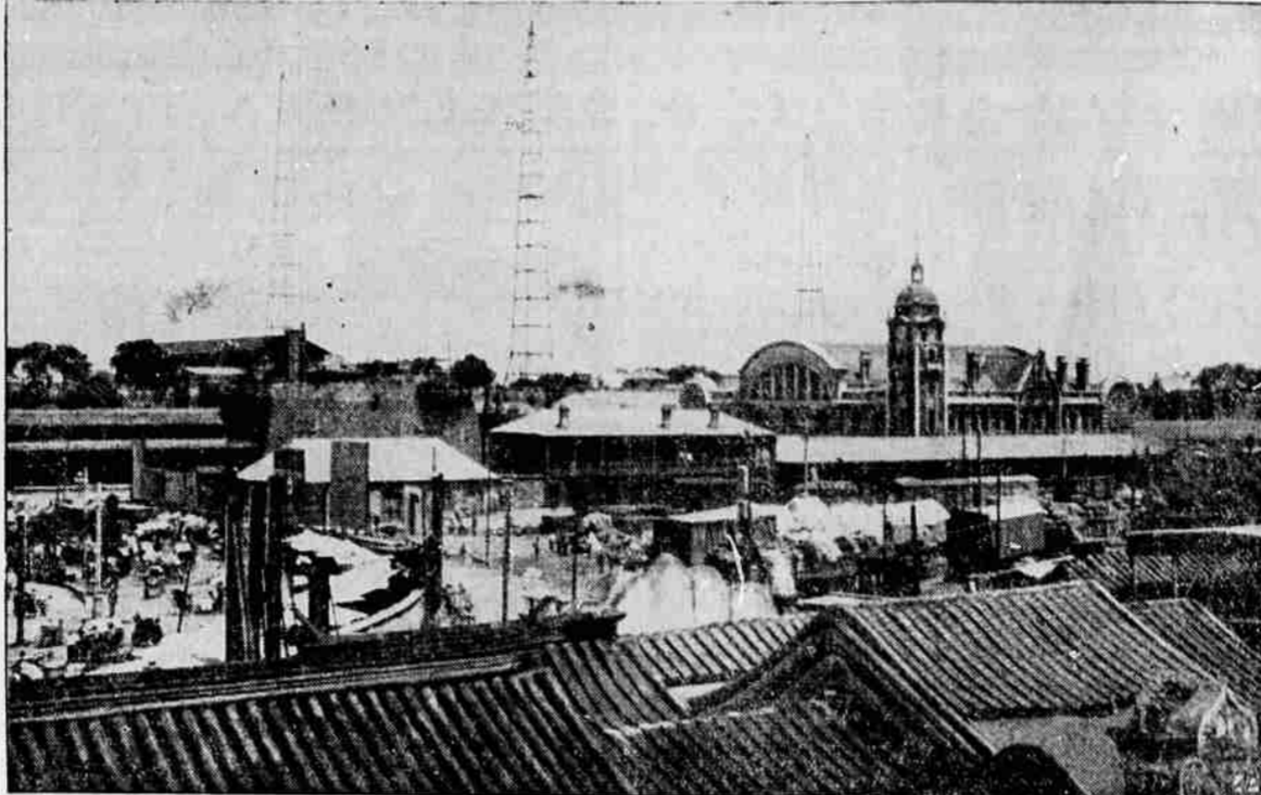
U. S. IN PEIPING. The wireless masts of the U. S. Marine radio station dominate the scene in the foreign legation quarter of Peiping, ancient Chinese city that now is the focal point of bitter clashes between Japanese and Chinese forces. At the right is the chief Peiping railroad terminal. Streams of troops from both Tokyo and Nanking were pouring into this trouble zone.
