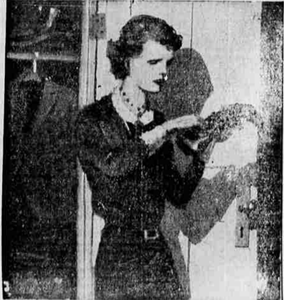
With a gasp, Kay saw a nail head missing.
