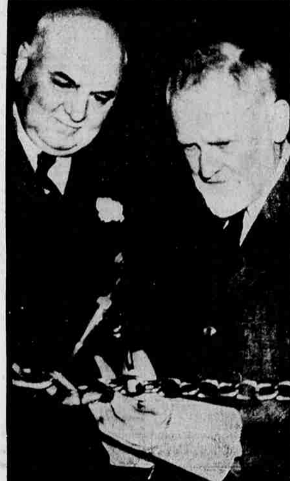
Frank P. Doyle (right) director of the Golden Gate Bridge and Highway District, and treasurer of the Redwood Empire Association is shown practicing the cutting of the chain, which will break the barrier of the Golden Gate Bridge on May 28. Mayor Angelo J. Rossi of San Francisco, who will also participate in the chain-cutting ceremony, is an interested spectator. The chain will be cut in three lengths by Doyle, Mayor Rossi and William P. Filmer, president of the bridge district, as a feature of the Golden Gate Bridge Fiesta.
