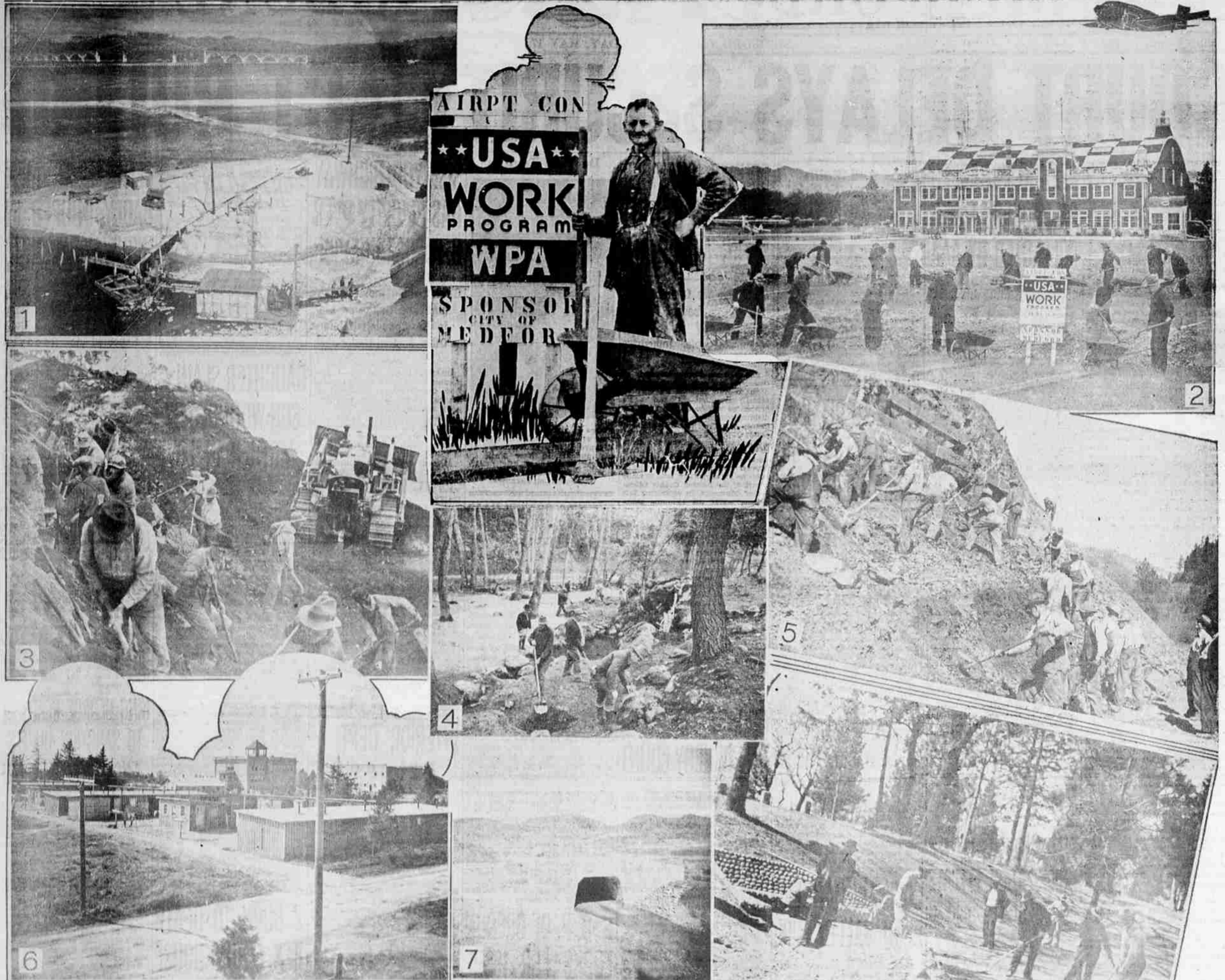
(1) View of the North Bend airport, WPA Project 695, showing dredge in the foreground pumping sand to raise the elevation of the field. The beautiful new Coos Bay bridge, completed during 1936, is shown in the background. (2) WPA workmen installing a drainage system in Medford's fine municipal airport with the hangar building painted by WPA crew in the background. Medford's airport improvement program is being conducted under WPA Project 1021. (3) Road construction in Josephine County was undertaken as a part of the WPA program for that area. This photograph shows workmen engaged in construction of the Merlin-Gallice section on the banks of beautiful Rogue River, a part of WPA Project 290-A. (4) The beautification of and addition of new facilities for Luthia Park in Ashland is another WPA undertaking. This is Project 1352. (5) When a disastrous forest fire almost wiped out the coast city of Bandon in the fall of 1936, the task of providing temporary shelters, hospital, city hall and rehabilitation of utilities was undertaken by the WPA. The accompanying photograph shows a portion of this housing program which is listed in WPA files as Project 1167. (7) A partial view of a 300 foot reinforced concrete culvert at the municipal airport of Roseburg. Improvement of this airport, Project 1175, is another WPA activity in southwestern Oregon. (8) The expansion and beautification of the Grants Pass municipal park is WPA Project 1235. This photograph shows a glimpse of workmen busy on this improvement work. (9) Glimpse of WPA workmen engaged in opening up Commercial Avenue, a two elevation street in the city of Marshfield. This Project 1230 is another evidence of the cooperation of the Works Progress Administration with municipalities of southwestern Oregon
