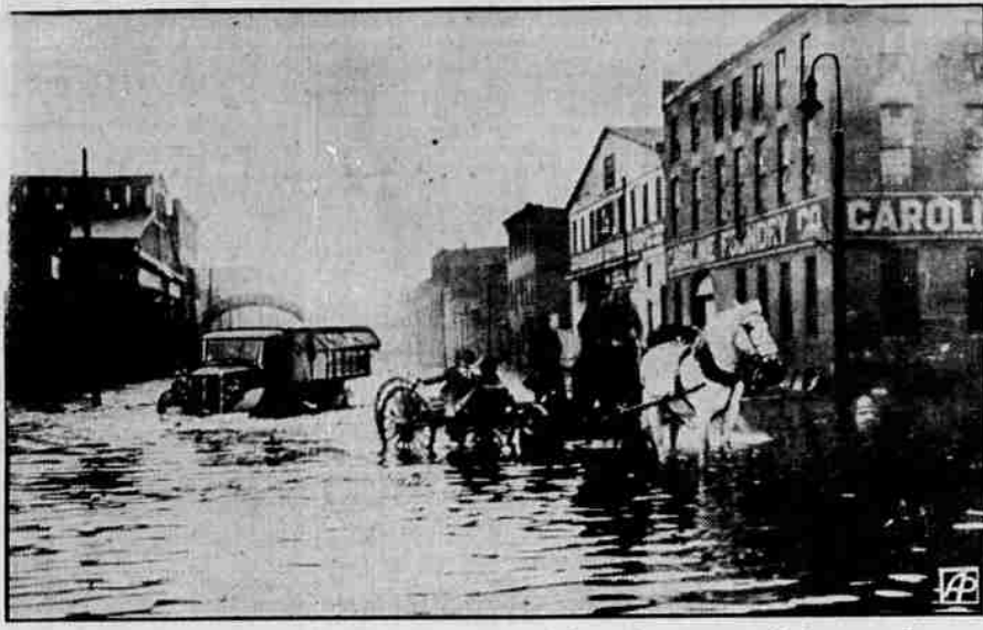
Horse-drawn wagons were pressed into service in Baltimore to remove goods from warehouses flooded by a high tide which surged into the harbor. The buildings shown here are several hundred feet from the water front in the industrial district.
