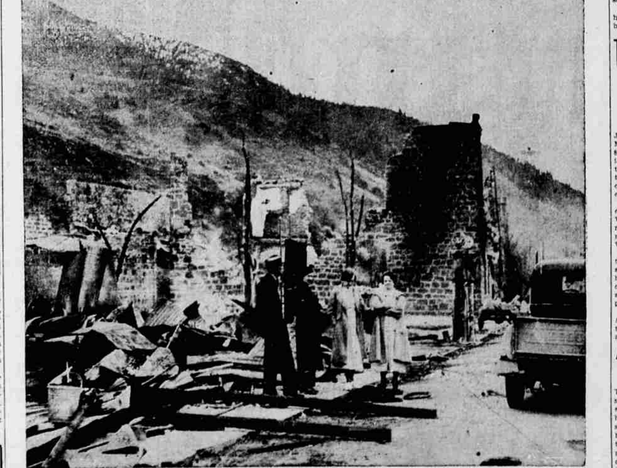
The business district of Canyon City, historic mining community of early days in Oregon, was virtually devoured by fire breaking out Monday night and burning until Tuesday morning. Residents are shown here surveying a section of the smoldering ruins after the exhausting battle against the flames. Fifteen business buildings were lost and several homes destroyed. Damage was estimated at about $100,000. Canyon City has about 350 residents. (Associated Press Photo.)
