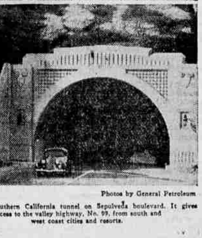
ABOVE—Southern California tunnel on Sepulveda boulevard. It gives access to the valley highway, No. 99, from south and west coast cities and resorts.
