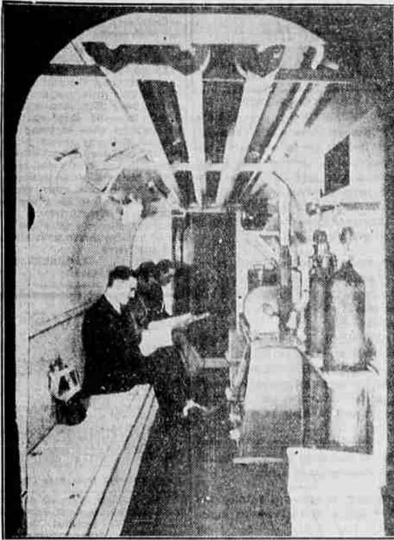
Great Britain's preparedness campaign against "the next war" has resulted in London's first gas and bomb-proof office building. The unique "war-conditioning" was installed as an experiment in the three-story establishment of its inventor, where 50 persons work. An interior view of the shelter, built in the basement, is shown here. It is equipped with air-lock doors and gas-filtered ventilation. (Associated Press Photo)
