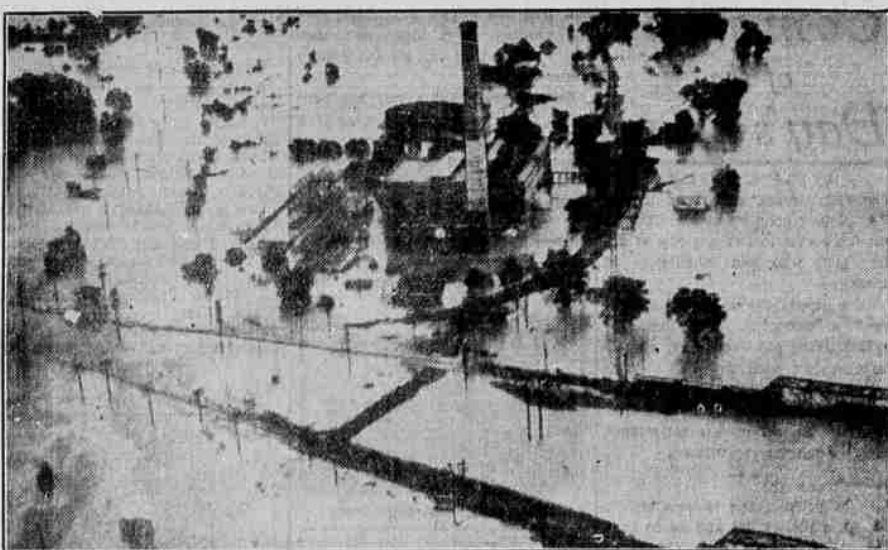
This picture shows the extent of a flood when the Brazos river broke over its banks and swept over a large section of Waco, Texas. The city power plant here was flooded, and water rushed over the approaches to two railroad bridges in the foreground. Two thousand were homeless. (Associated Press Photo)
