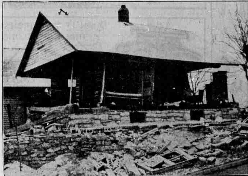
This was the freak result of an explosion, apparently caused by an accumulation of gas, at the home of Mr. and Mrs. Ed Burris at Kansas City. Although the blast blew out all four walls of the home, it left the roof intact, supported by the room partitions. Neither of the occupants was seriously hurt. (Associated Press Photo)
