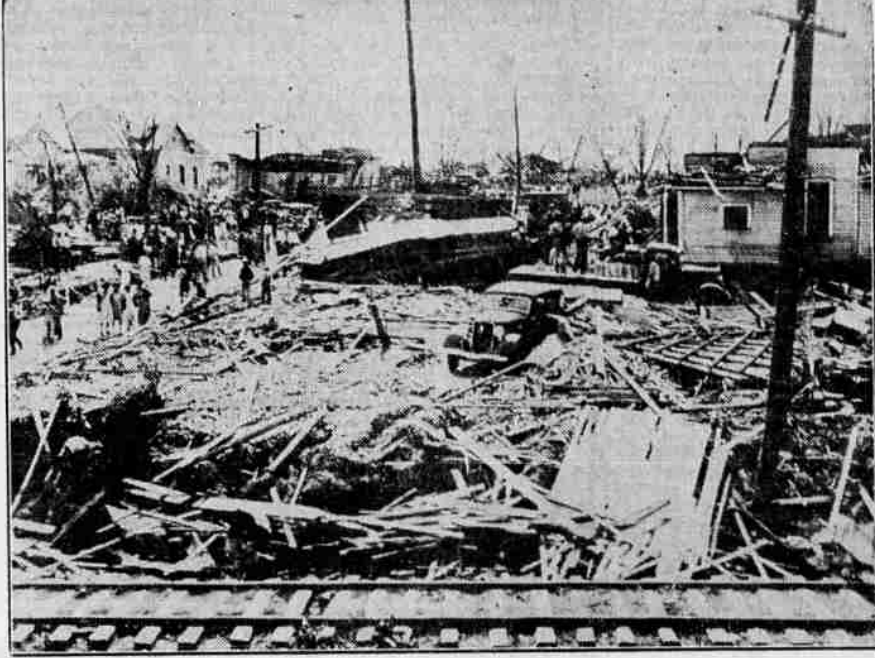
A devastating tornado that twisted through Cordele, Ga., left the city largely a scene of heaped debris and widespread suffering. Eighteen persons were killed, and many were homeless as hundreds of homes lay in ruins. This general scene of the splintered wreckage gives a vivid picture of the damage done by the storm. Four men were killed in a store, whose wreckage may be seen in the center of the picture next to the street. At least 39 were killed in storms in various southern communities. (Associated Press Photo)
