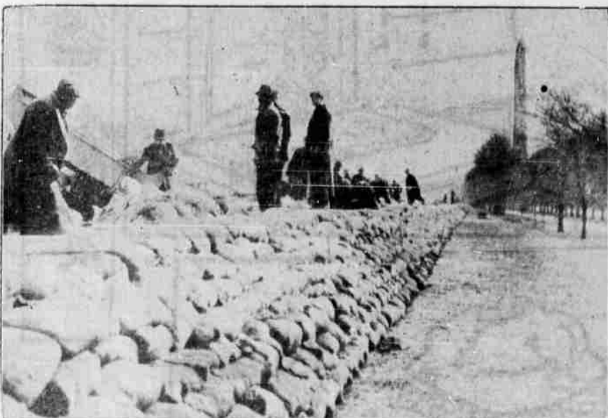
As the flood waters of the Potomac river rushed on to Washington, D. C., relief workers were ordered to rush the completion of a sand bag dike to protect the foundations of the Washington Monument and the Lincoln Memorial from the overflow. The Washington Monument may be seen in the right background. (Associated Press Photo)
