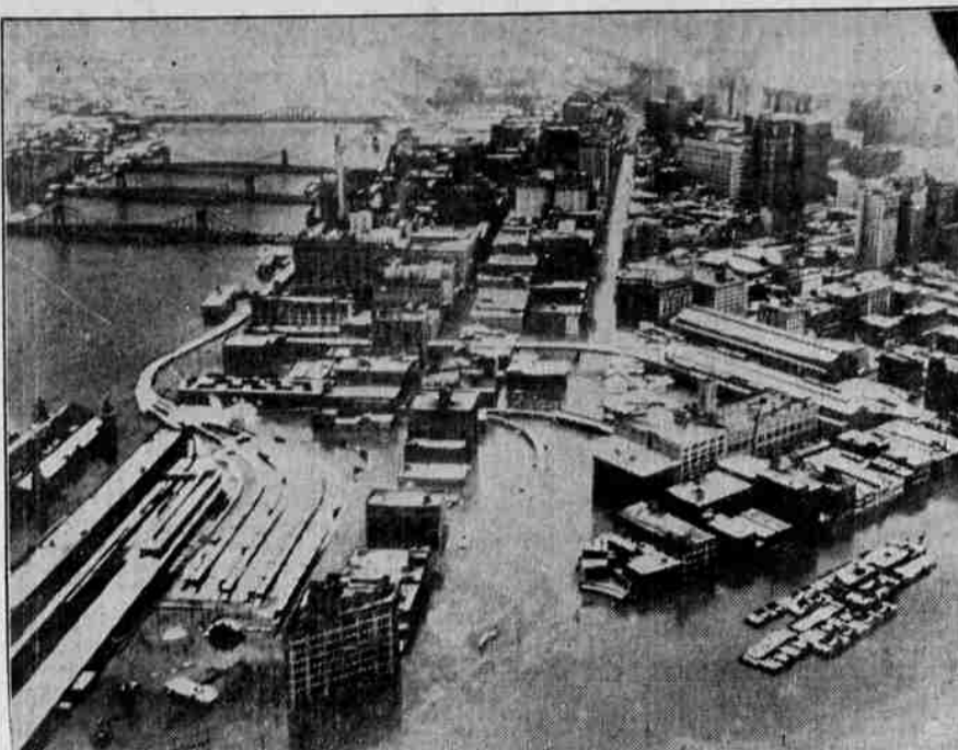
This graphic aerial photograph shows how the famous "golden triangle" business center of Pittsburgh, Pa., was inundated by the turbulent waters of two rivers near the junction that forms the Ohio river. Receding of the water left the section covered with slime, and national guardmen ruled the district under martial law to prevent possible looting. At least six persons were killed in Pittsburgh, and damage of more than $25,000,000 done by the flood, worst in the city's history. (Associated Press Photo)
