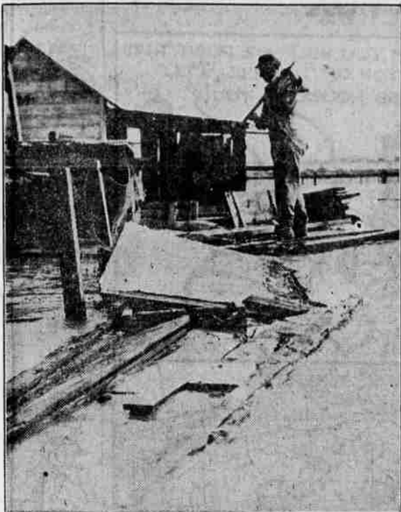
A resident of an outer district of Stockton, Calif., is shown here working from a makeshift raft to remove floating timber pile up against his home when flood waters from Bear creek flowed more than two feet deep through some of the residences in the district after continued storms. (Associated Press Photo)
