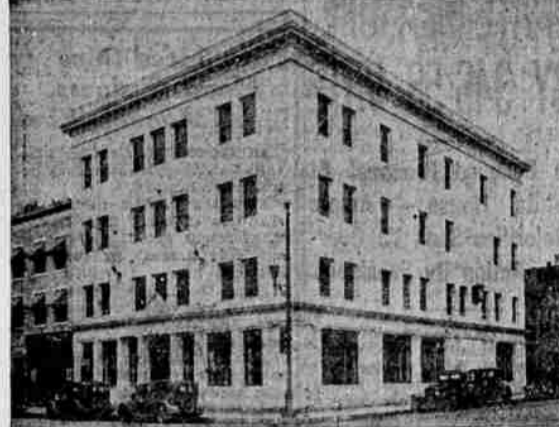
Above is shown "before and after" views of a Massachusetts bank which underwent an exterior modernization recently. Several improvements were made in the plan and general appearance of the structure. The entire exterior was faced with cut limestone, and the former outmoded appearance of the building is now supplanted by an atmosphere of modern dignity. Such modernization projects may be carried out with funds obtained under the Modernization Credit Plan of the Federal Housing Administration. Full information may be obtained at any local office or by writing the Federal Housing Administration, Washington, D. C.
