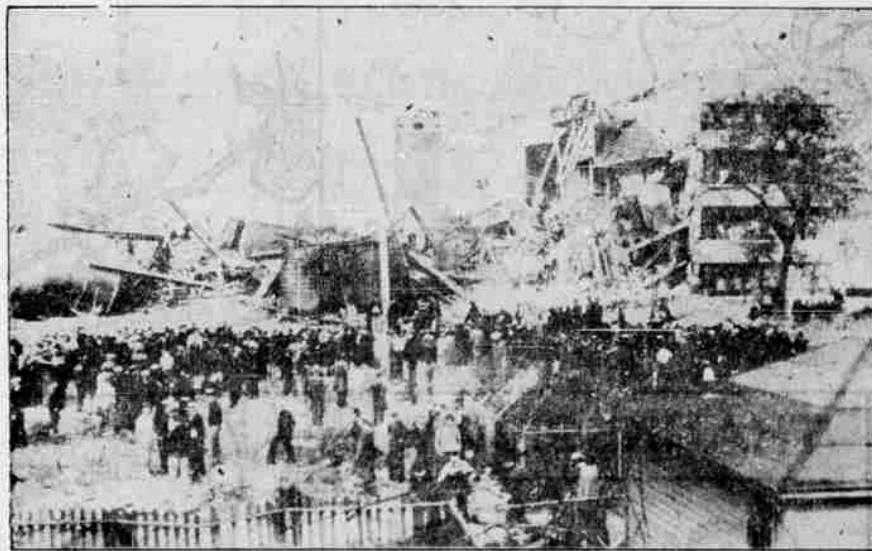
At least seven were killed and more than 30 believed badly hurt when an explosion tore apart a Chicago paint factory. Damage done to the building is shown above. (Associated Press Photo)
