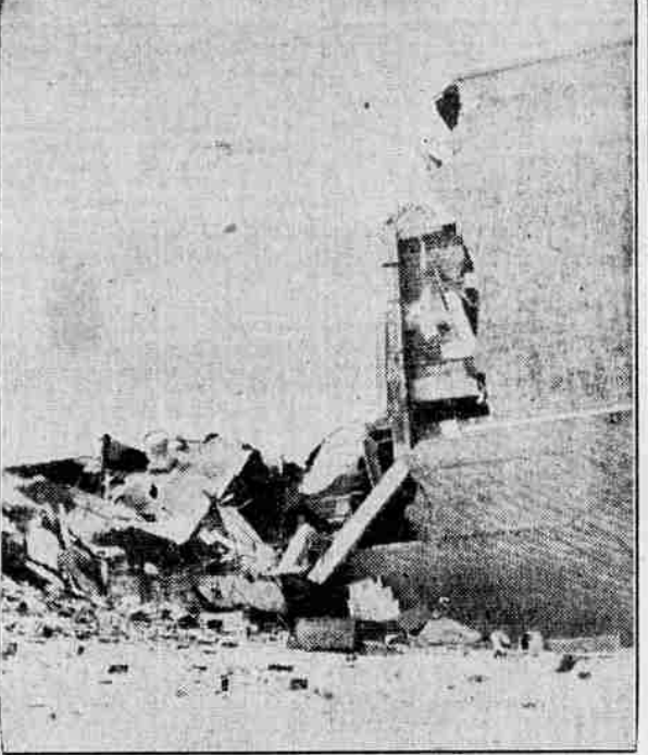
This is the wreckage of new $500,000 high school which crumpled and sent workmen fleeing when the earth quaked in the second strongest of approximately 500 earthquakes during 19 days in Helena, Mont. (Associated Press Photo)
