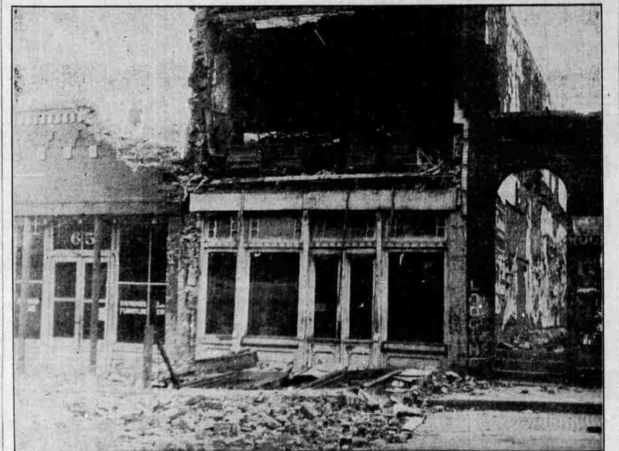
Dave Harris, a negro, was crushed to death when this building collapsed in Helena, Mont. One other person was known to be dead and nearly a score injured in the severe earth shocks which hit the Montana capital. This picture, rushed to The Mail Tribune by The Associated Press, gives a vivid account of the damage done by the tremor. (Associated Press Photo.)
