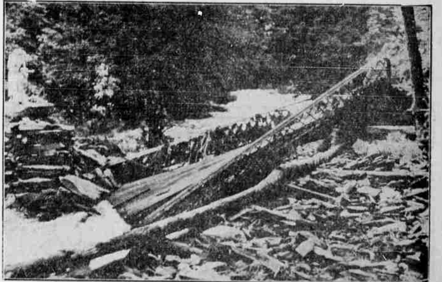
One of the many bridges washed out by a cloudburst which swept through southern tier counties of upstate New York, taking at least 36 lives, causing property damage of an estimated $10,000,000 and rendering hundreds homeless. This bridge was washed out near Woodstock. (Associated Press Photo)
