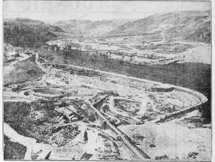
The world's largest conveyor system, being used in the construction of Grand Coulee dam, can be seen in the foreground of this picture. Over this system of belts the material being taken from the old river bed to Rattlesnake canyon about a mile and a half away and 500 feet above the bottom of the excavation. This general view of the excavation in southeastern Washington at the dam shows the Mason City contractor's camp in the background. (Associated Press Photo)
