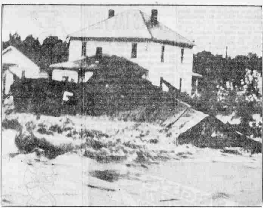
A flood which struck Lancaster, Ohio, is shown in the picture snapped by an amateur photographer just after it had battered down the home in foreground occupied by William Johnson. Neighbors rescued the family. Damage in the area brought an estimate of $2,000,000 as hundreds were made homeless. (From Associated Press)
