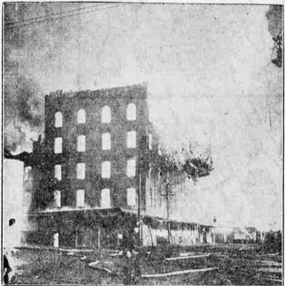
Damage estimated in excess of $400,000 was done when flames destroyed the Taylor Milling Company plant at Stockton, Calif. A section of the wall is shown plunging downward during the height of the fire. One fireman was injured by falling bricks. (Associated Press Photo)
