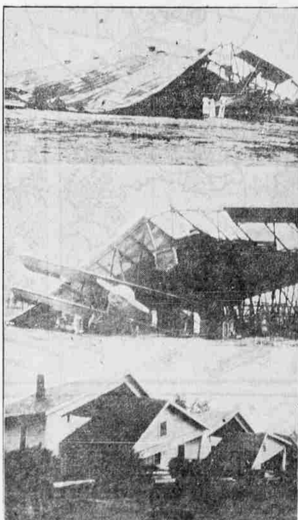
A sudden windstorm which struck Texarkana, Tex., and vicinity left four dead and several injured. Damage done to the airport is pictured in the top and middle. Several residences were battered down by terrific winds. (Associated Press Photo)
