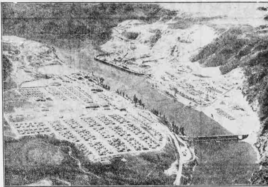
The great reclamation project of the Pacific northwest, the Grand Coulee dam site in southeastern Washington, is shown in this new aerial picture. It has been a busy place since construction started two years ago. The town on the left bank of the Columbia River is Mason City, built by the contractors. Across the city is Engineer's City, a government development. The west cofferdam, 3000 feet long is just above the latter. (Associated Press Photo)
