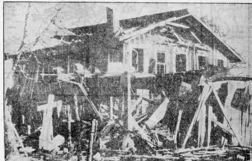
A terrific explosion of 250 kegs of blasting powder and 20 cases of dynamite nearly destroyed Helenwood, Tenn. Fifty homes and buildings were destroyed or damaged, seven persons injured and 75 made homeless by the blast. This picture is typical of the destruction caused. (Associated Press Photo)
