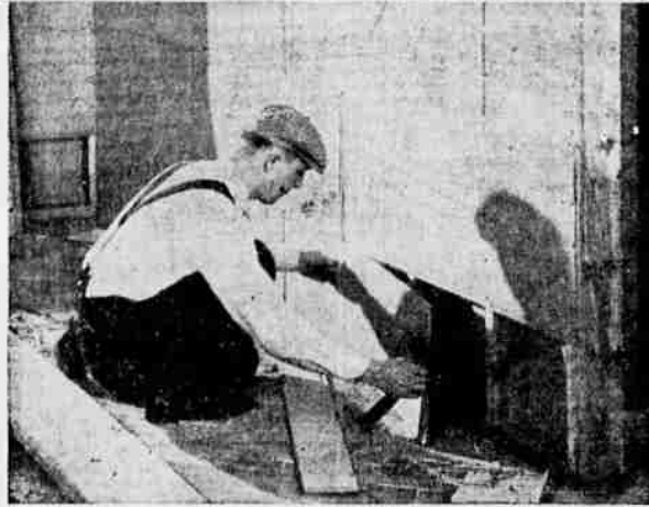
Transformation of cellar into attractive playroom and den made with insulating board (above), combines decorative, structural, insulating and acoustic improvements. Similar methods of improvement are possible with plaster on lath, plywood or insulating board. Below is shown a workman applying material.
