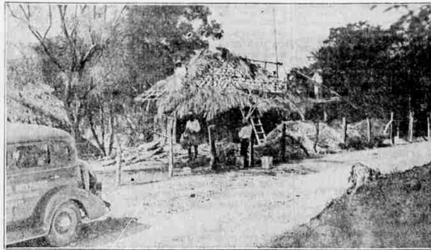
Beginning almost at the American border and extending to Mexico City, thatch huts are common dwelling places of the average Mexican farm worker. In the palm country, the huts, like the one pictured, are erected of saplings and roofed and walled with palm leaves, making a cool rainproof dwelling. The pathfinding car passed thousands of such homes en route to Mexico City on the Pan American highway.
