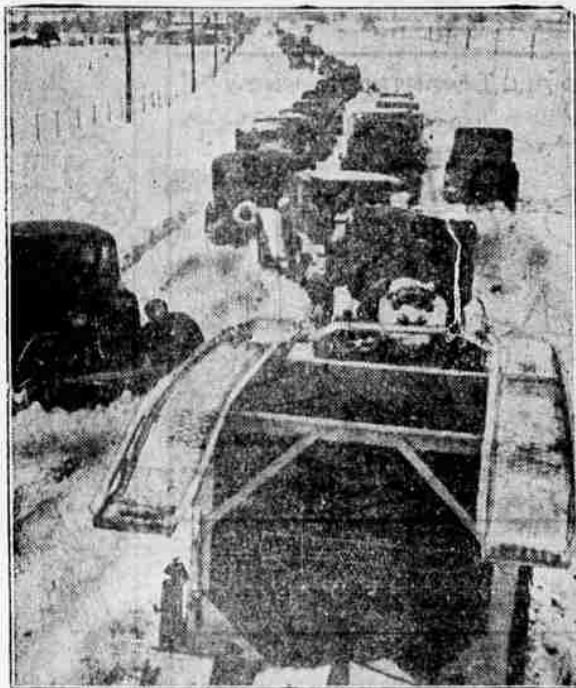
A typical mid-winter snowstorm arrived several months ahead of schedule in Missouri and tied up more than a thousand motorists on U. S. Highway No. 66, a few miles east of Springfield, Mo., before snow plows could be rushed to the scene to open the road. Most of the stranded motorists sought aid at the nearby town of Strafford which has a population of only 125. (Associated Press Photo)
