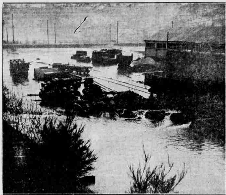
The railroad freight yards in Seattle, Wash., are shown covered by flood waters following slides in the mountains east of the city and floods in the lowlands. Seattle was cut off from the east by rail and highway by the mounting waters. (Associated Press Photo)
