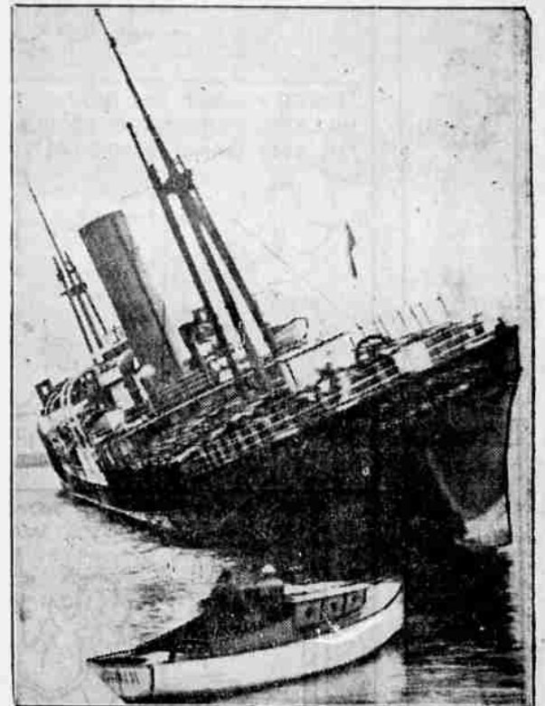
A bursting ballast tank while the vessel was 200 miles off Cape Flattery, Wash., on her way to the orient with a lumber cargo almost spelled disaster to the Britisher freighter Capte Ortegal. Listing badly, the ship was able to make Victoria, B. C., unaided and is shown on arrival. (Associated Press Photo)
