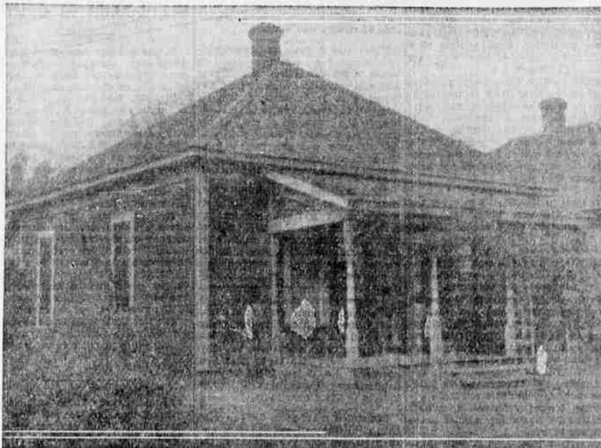
In co-operation with the National Housing Act, the Medford Federal Savings and Loan Association sponsored this little, small-family home at 1506 West Main street. Top, the home after the economical program had been completed and ready for public inspection today. Bottom: The little house as it appeared before modernizing. Home labor and materials were employed and local firms have co-operated in furnishing this attractive little residence.
