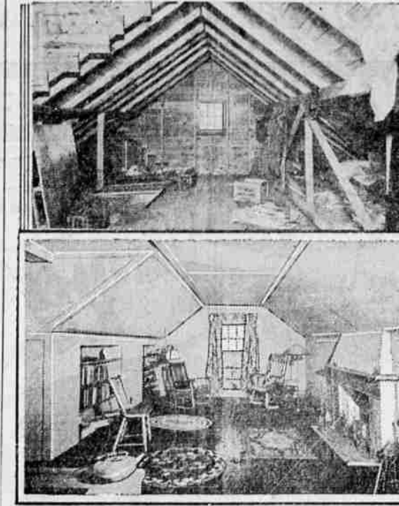
A little wallboard, some appropriate furnishings, and some ingenuity converted the wasted attic space shown in the upper picture into the cozy room revealed in the lower illustration.
