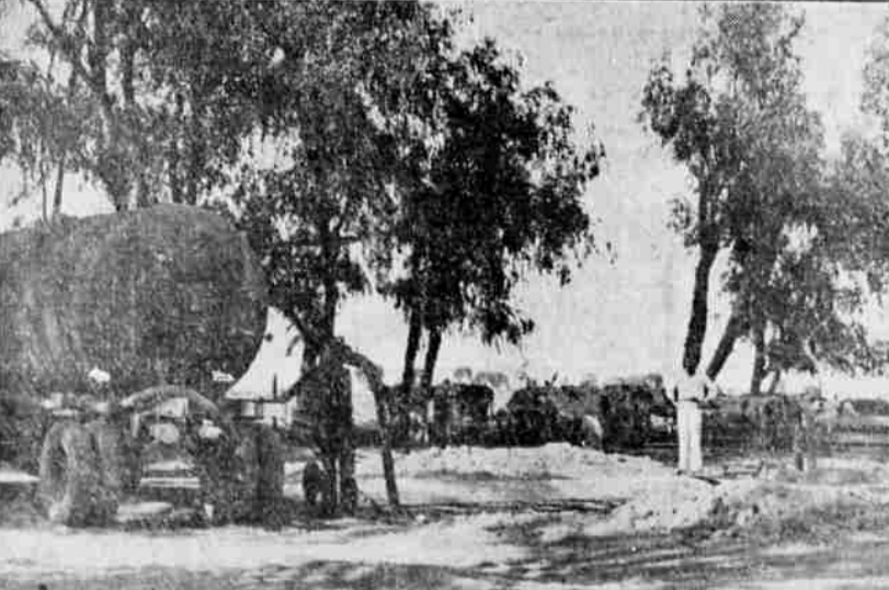
The scarcity of water in Imperial Valley, Cal., was so acute that dairy and beef cattle were watered by tank trucks, operated by the SERRA. A truck is shown filling an emergency cement tank buried in the ground. The present drought is expected to be the last in the valley, as the completion of Boulder dam will assure ample water. (Associated Press Photo)
