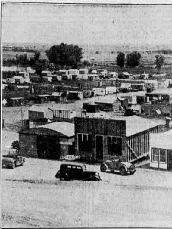
This village is New Deal, the nation's newest community. It has sprung up at the site of the Fort Peck dam in Montana. The dam to be built across the Missouri river at this point is a public works project, and is to be second in size only to Boulder dam. (Associated Press Photo)
