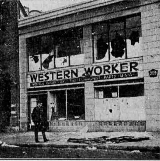
The entrance to the headquarters of the Western Worker as it looked after a group of what was termed "young vigilantes" descended upon the place in a series of raids upon asserted radical gathering places in San Francisco during the general strike. The crowd had disappeared by the time police appeared in answer to a riot call. (Associated Press Photo)
