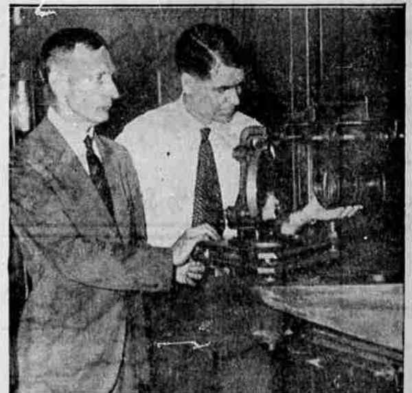
A new camera built in the basement of the Commerce building in Washington for the United States coast and geodetic survey weighs 15 tons, cost $15,240 and makes pictures 50 inches square. Capt. R. S. Patton (left), director of the survey, and Lieut. O. S. Reading, the designer, are shown examining the lens of the camera, which was developed to reproduce maps and charts cheaply and accurately. (Associated Press Photo)
