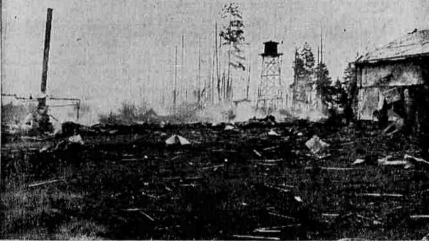
The devastated plant of the J. A. Dem powder plant on Hawks Prairie, six miles east of Olympia, shortly after the terrific explosion June 27 that killed ten persons and injured six. The upper view shows what was left of the chlorate and mixing rooms, where the fire which led to the blast was believed to have started. The lower scene depicts a general view of the devastation.—(Associated Press Photos).
