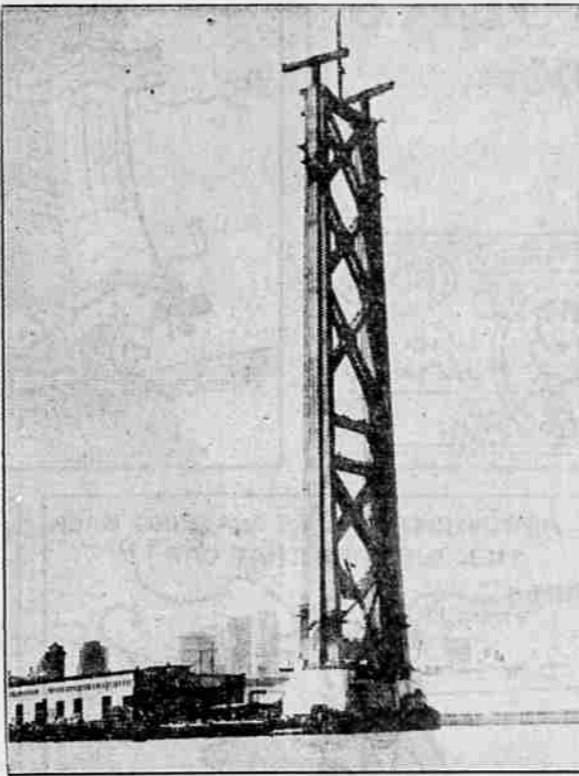
Towering high above the San Francisco waterfront, the principal tower of the San Francisco-Oakland bay bridge on the west side dwarfs the skyline of the city. The structure is almost complete, the saddles for huge cables remaining to be put in place. The steel structure looks like this to commuters coming from Oakland. (Associated Press Photo)
